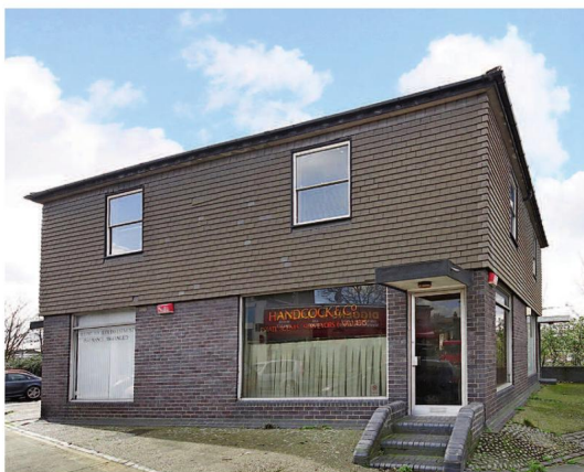
Delacourt Road, SE3 £2,083 PCM
